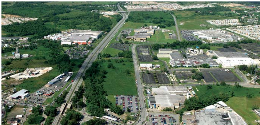
In the area of Las Piedras, a popular industrial district, Christiansen & Portela is offering an industrial facility for sale in Las Piedras Industrial Park.
